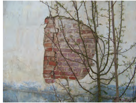
Figure 10. Places unclosed with walls of the historical window of Svēte palace (author's photo, 2004).
